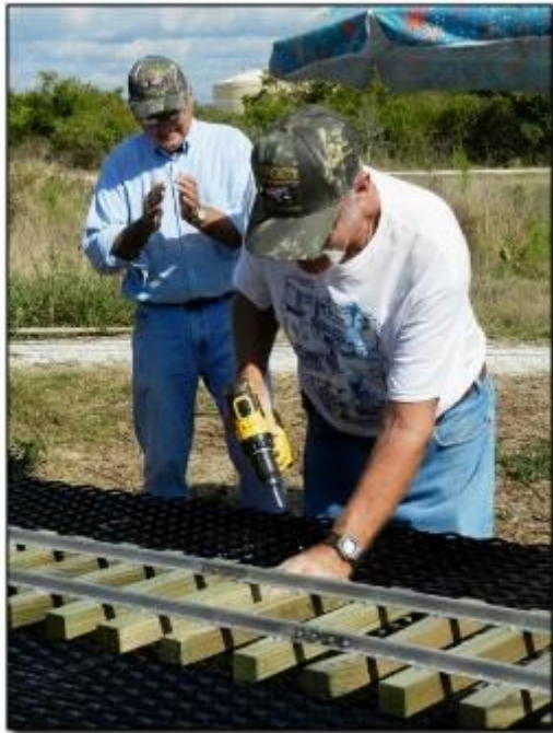
Tom Pfister installs the last screw; Richard Dobler in background
