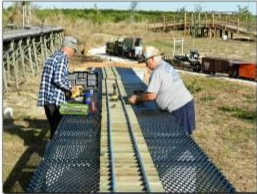
Here they are installing the final rail joiners
